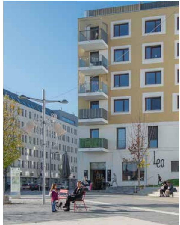
Public space with a high quality of sojourn at Hannah Arendt Platz. / Luzia Puiu © 3420AG
